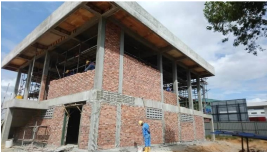
Electrical substation construction
