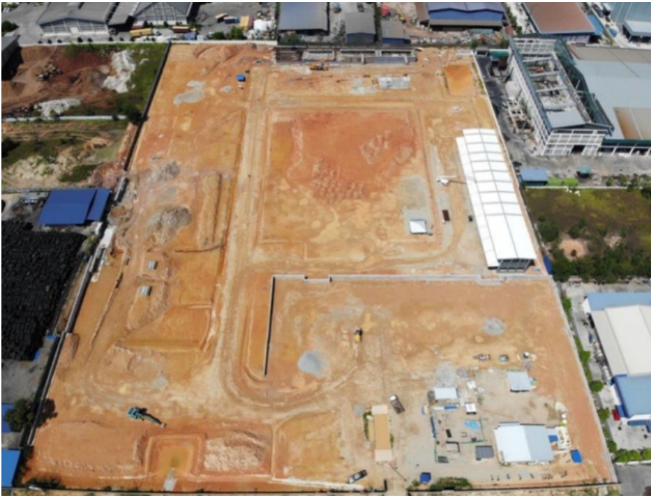
Overall site view showing construction progress at HPA Project site
