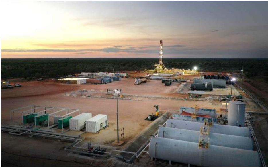
The Ungani Production Facility and NGD 405 rig at Ungani 6H development well location.
